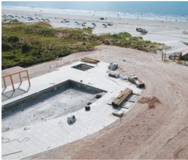
The pool, under construction at the Timbers Beach Club.
